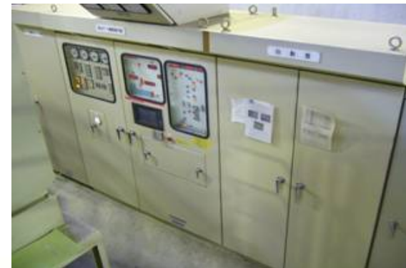
Control panel (The button used for moving the gate is located on the panel.)
