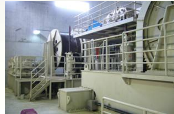
Winch (The gate is moved by controlling the wire rope.)
