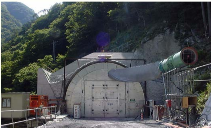
Soundproofing wall against blast
