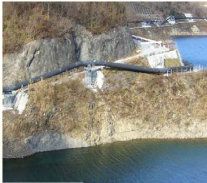
Steel water pipe channel section of the bypass pipe
