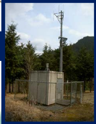
Hosokubo Rain Gauge Station
