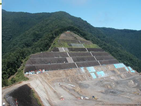
Excavating aggregate and replacing stored soil (during construction)
