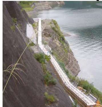
Prelining concrete section of the bypass pipe
